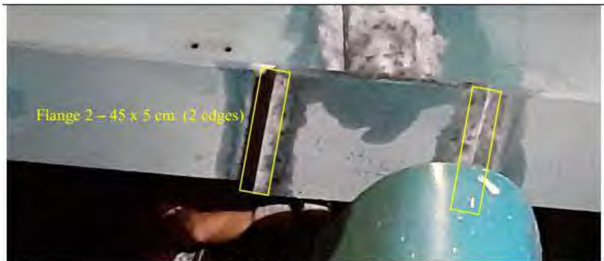
FIGURE 3: Item B – Flange 2 (opposite side to Flange 1) No relevant indication
